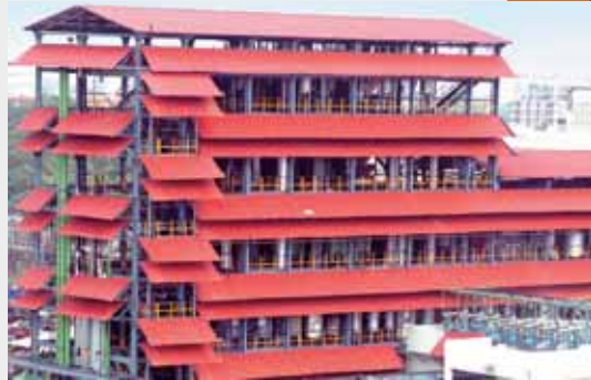
Multi Product plant at Surat
