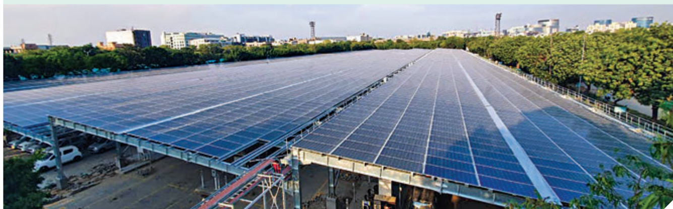
5 MWp carport style solar PV plant at the Gurugram facility
