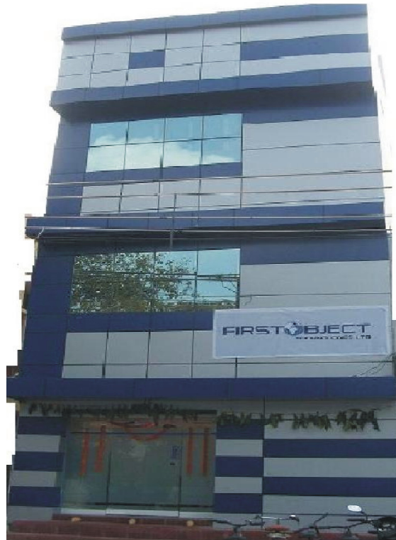
(inset : Original Picture of Firstobject Office at Kakinada)
