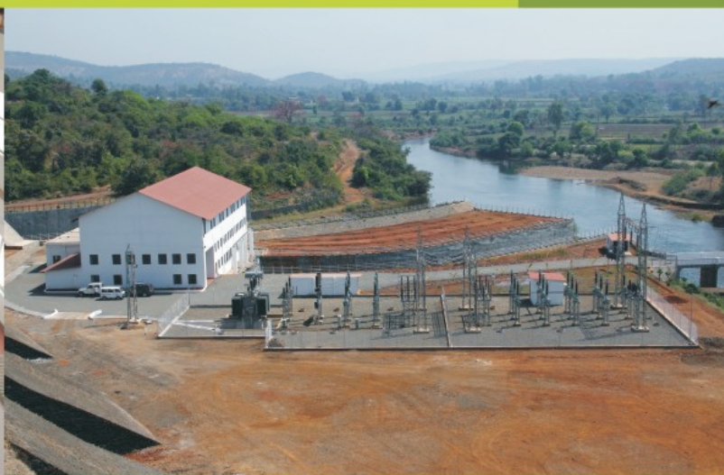
The Power House Building and the Electricity Grid
