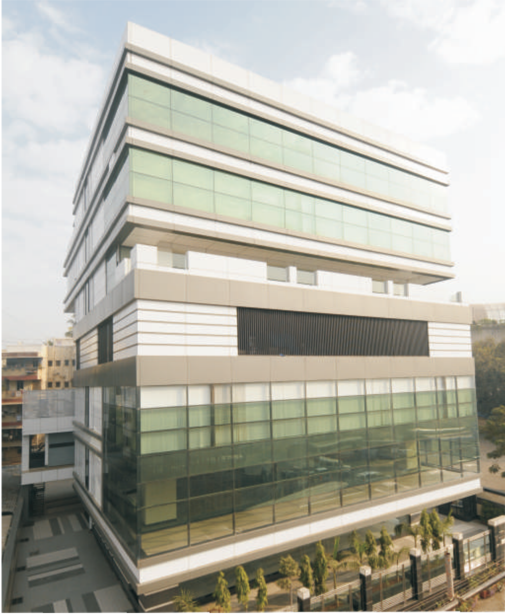
Completed Commercial Project
