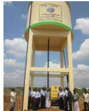
OVERHEAD WATER TANK PROVIDED TO VILLAGERS BY SANKARNAGAR WORKS
