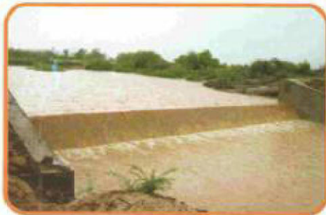
Check Dam, Village Sambhda, Tal : Lakhpat storage capacity 72 lacs litre.
