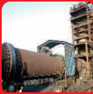
Coal Based DRI Plant
