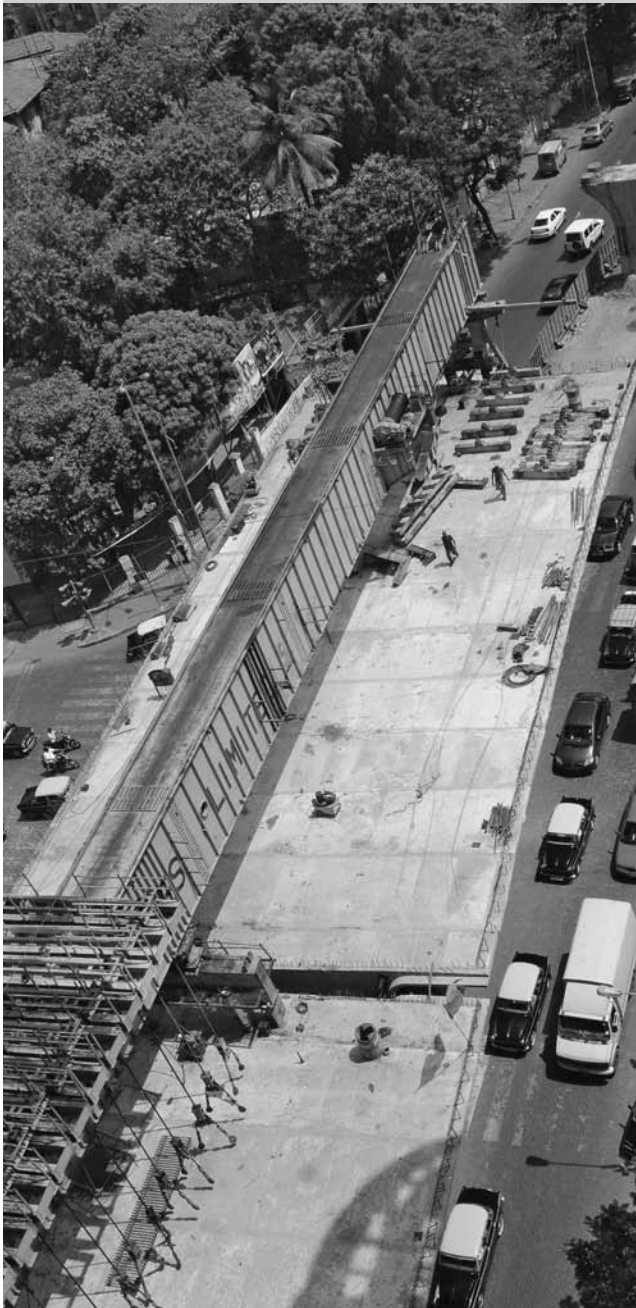
Metro Project - Mumbai
