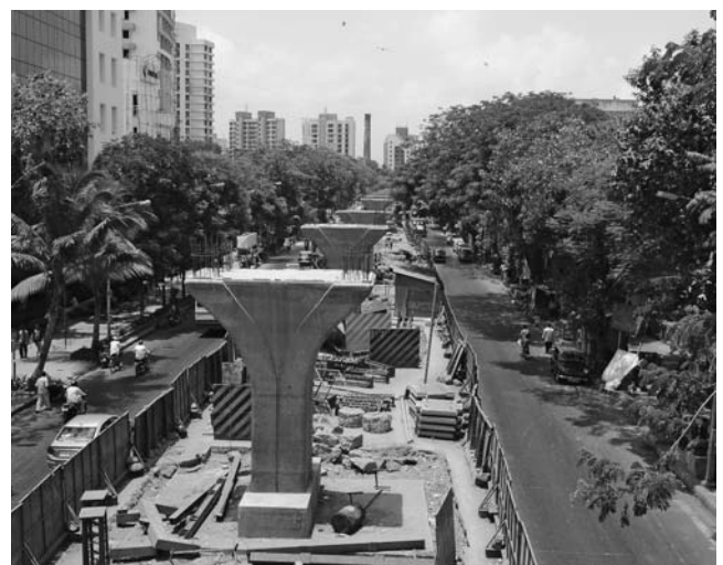
Flyover Construction at Guwahati, Assam
