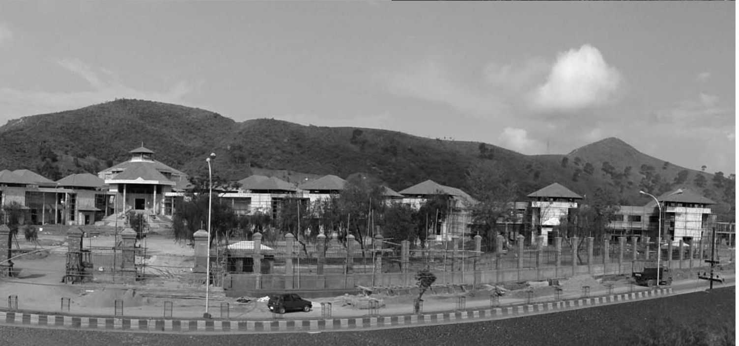
A Panoramic view of High Court Complex at Imphal - design & construction by Simplex
