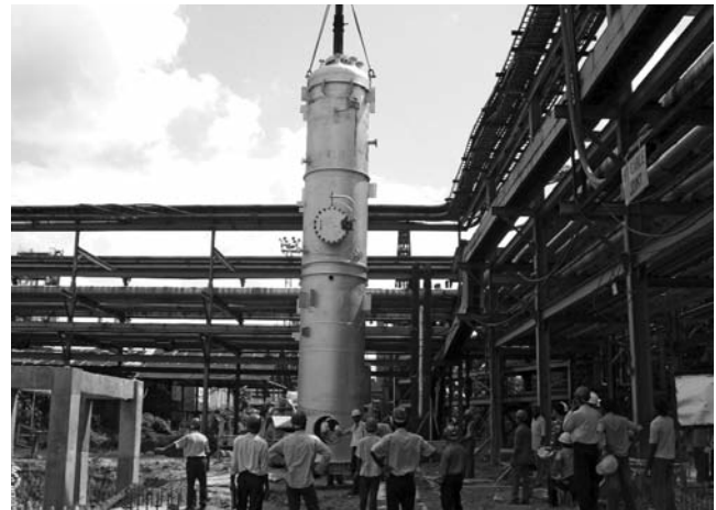
Equipment Erection 37-VV-013, IOCL Digboi, Assam
