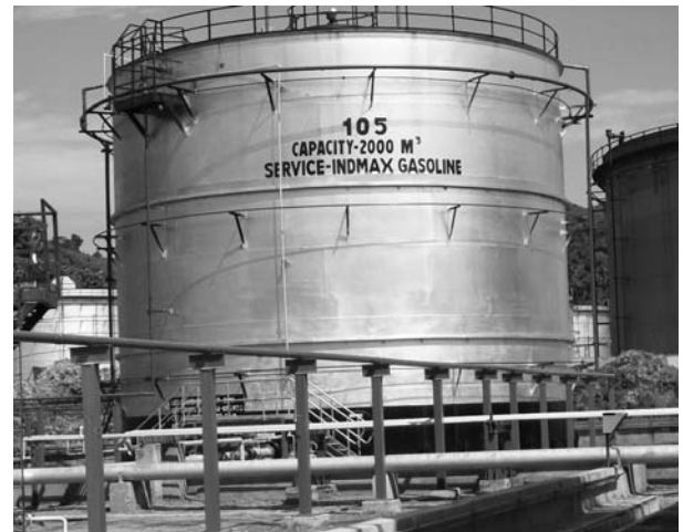
Heavy Gasolene Feed Tank for IOCL, Digboi, Assam
