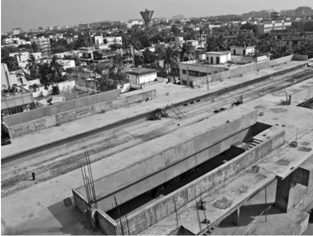
Elevated Station Building for East West Metro, Kolkata
