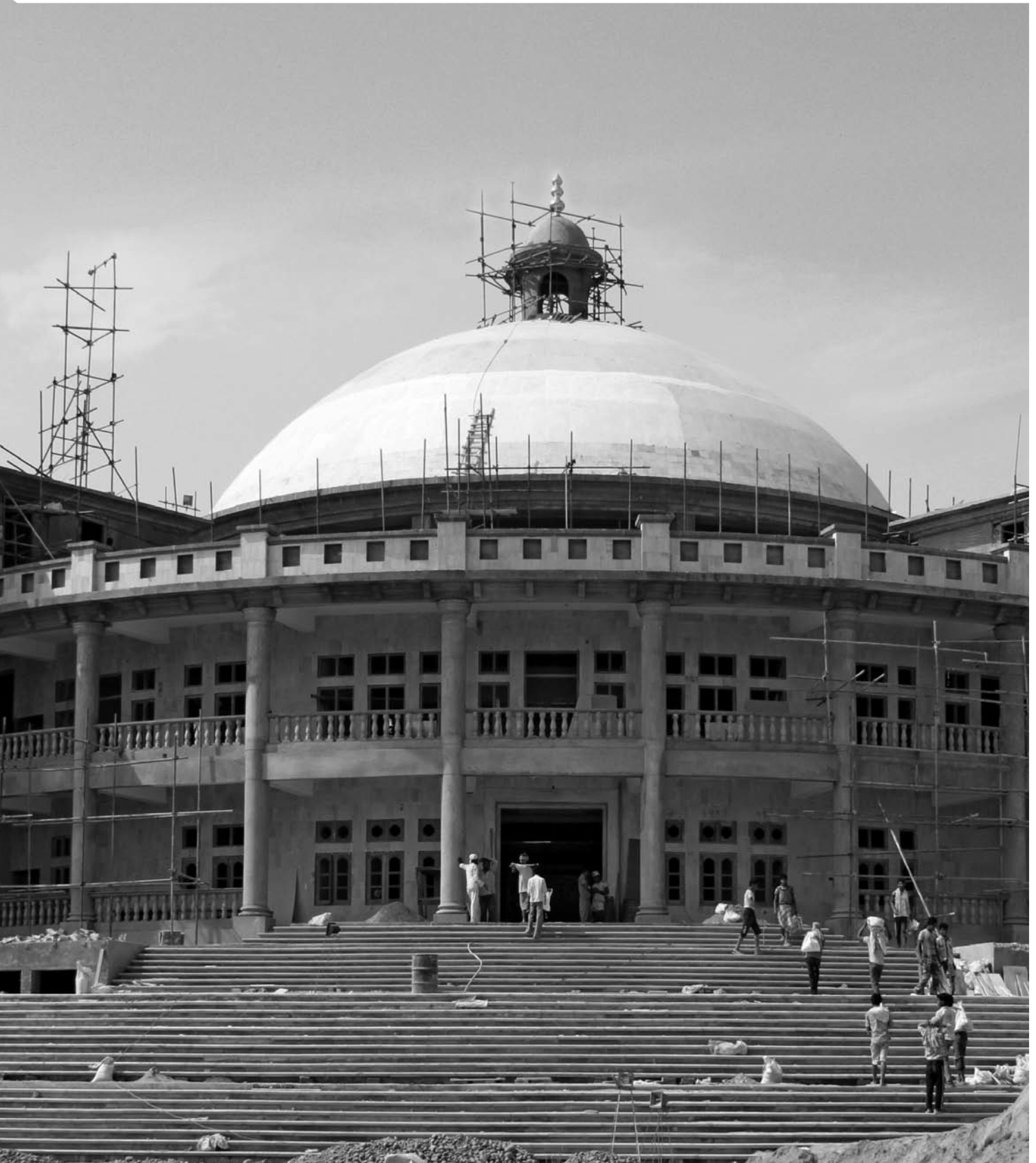
Design & Construction of Assembly Building at Imphal
