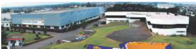
Menon Bearings plant at Kolhapur
