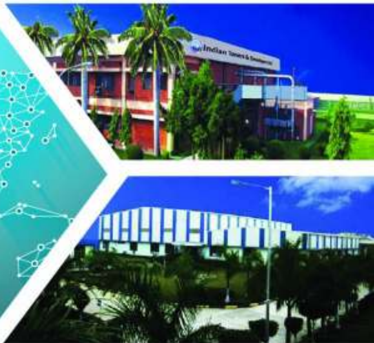
World-class Manufacturing Facilities
