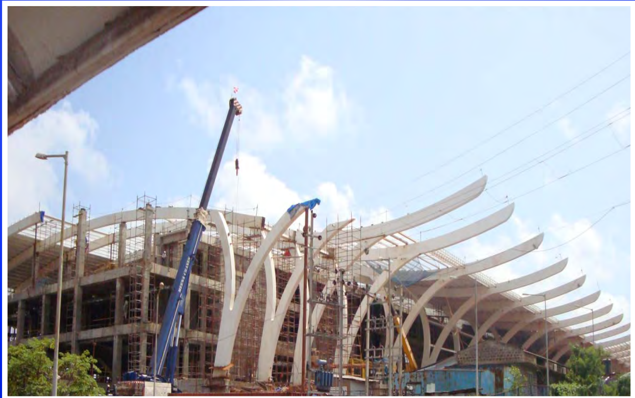
New Integrated Terminal under construction since May 2011 at Dabolim International Airport
