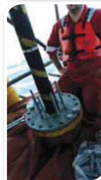
Composite power cable is being pulled through Hanger/hang off clamp
