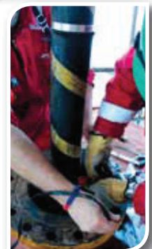
Composite power cable is being prepared for hang off
