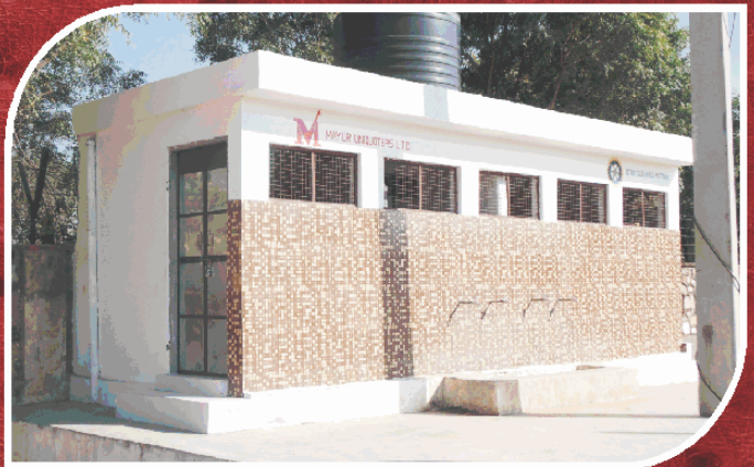
Constructed New Toilet (Apni Azadi)
