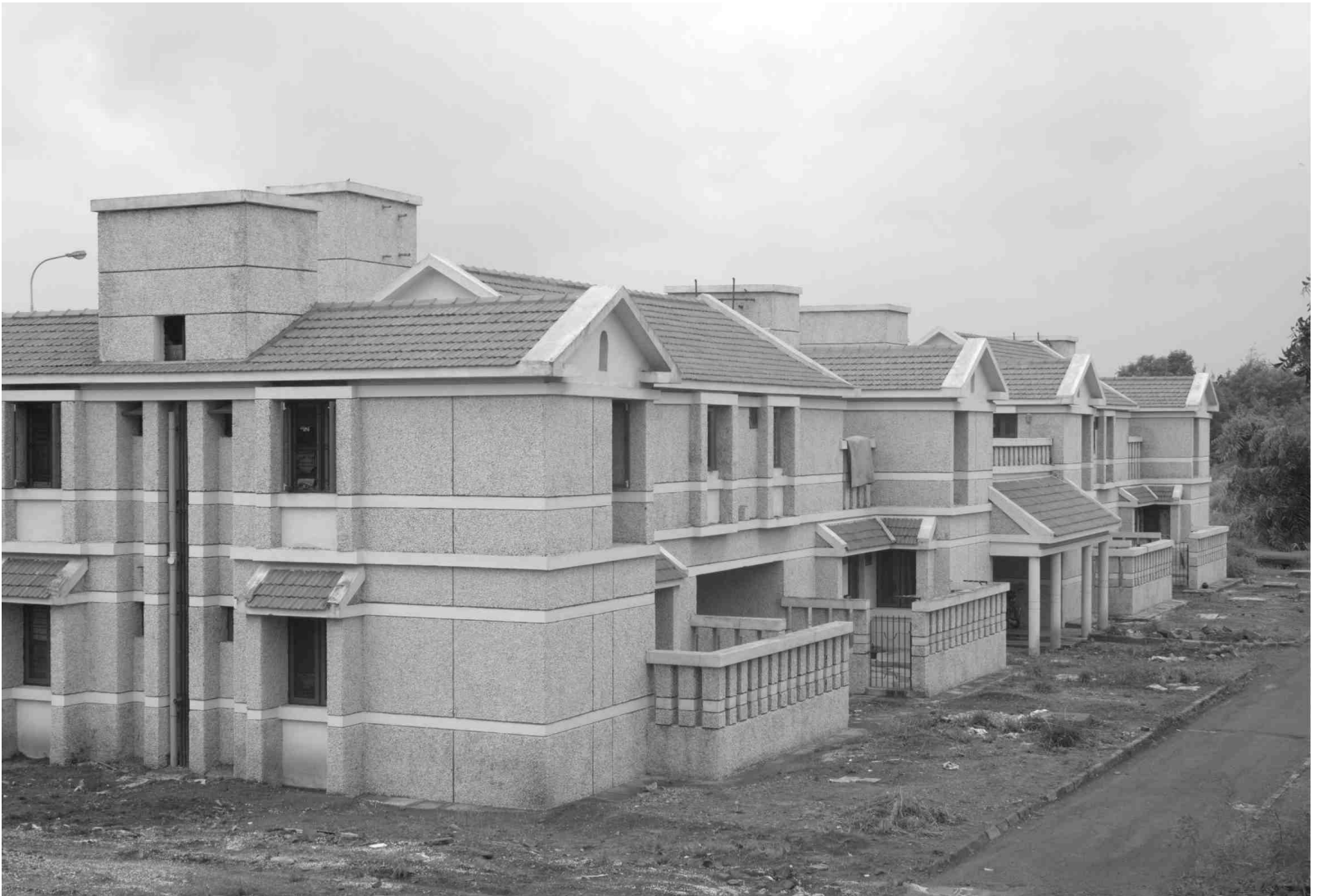
work as "GIPCL Township Expansion Work at Nani Naroli, Gujarat"
