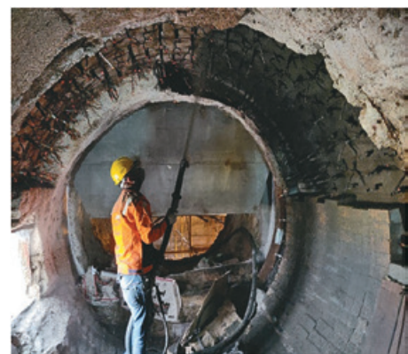
▲ DURAGUN application in progress in cement plant
