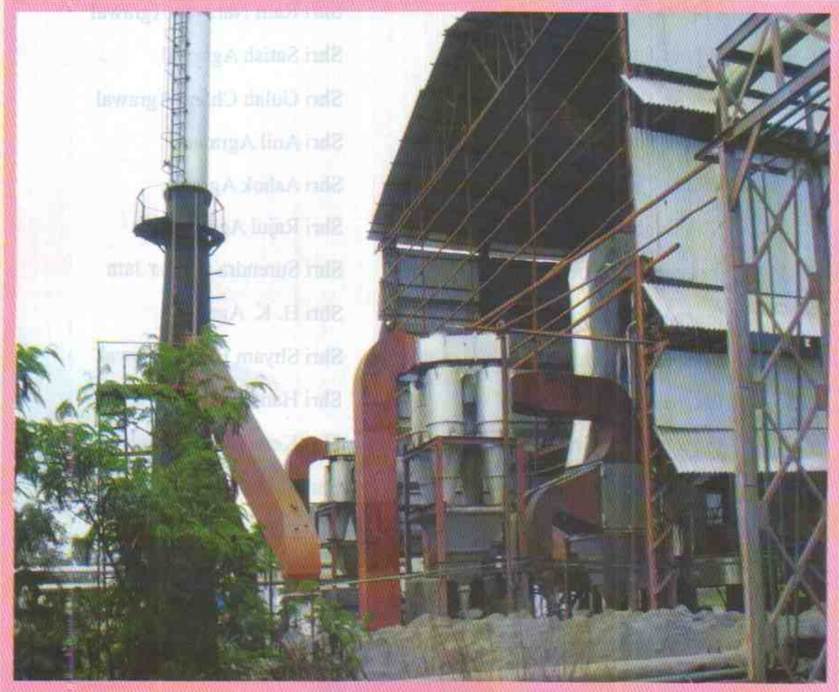
Solvent Extraction Plant at Mandideep
