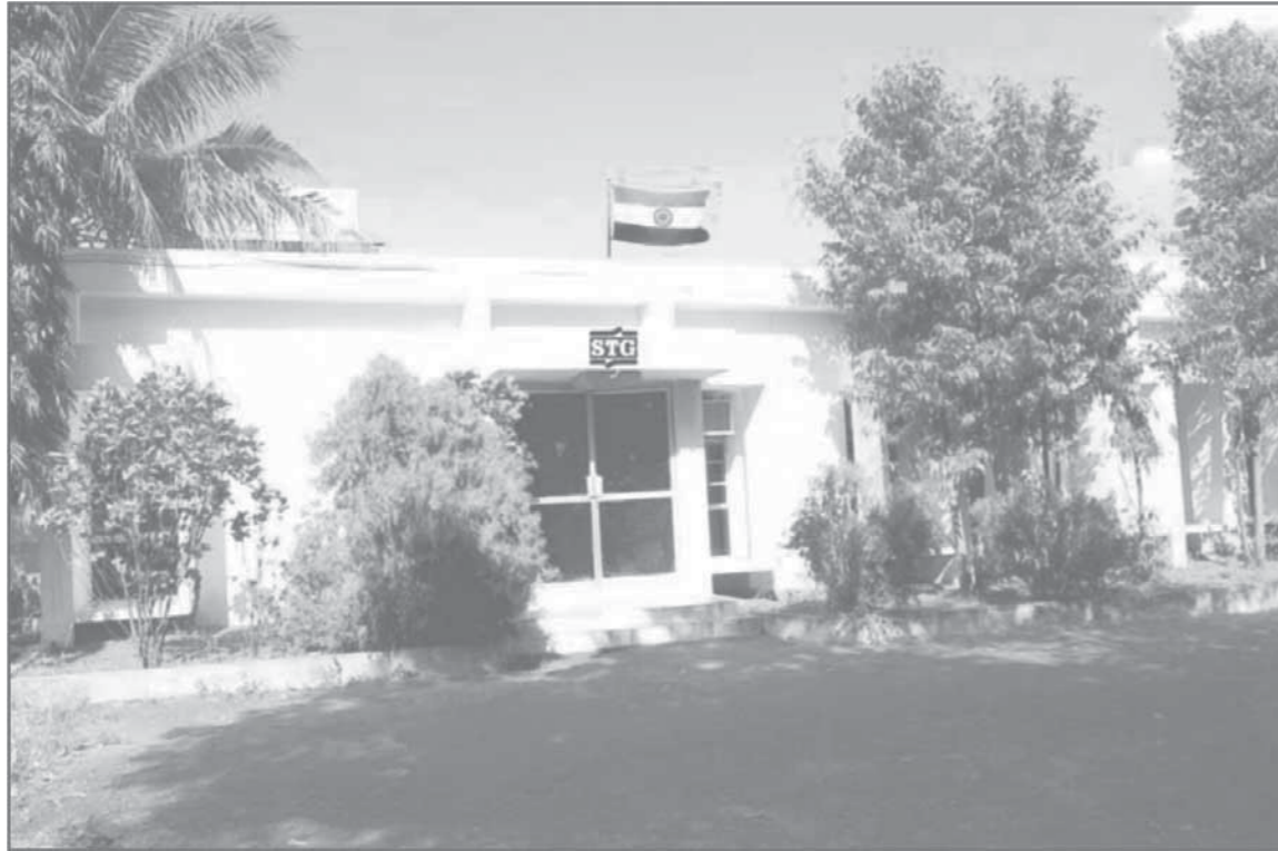
FRONT VIEW OF STG
