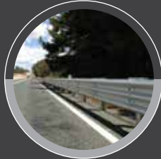
HIGHWAY GUARD RAILS
