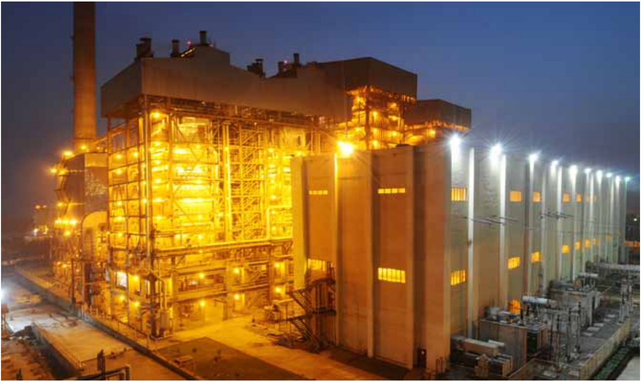
Night view of the 114MW Power Plant at Andhra Pradesh
