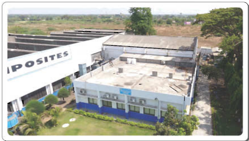
Technology center at Paithan
