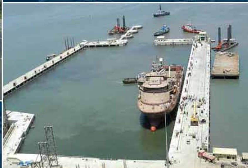
Wet Basin at Mumbai
