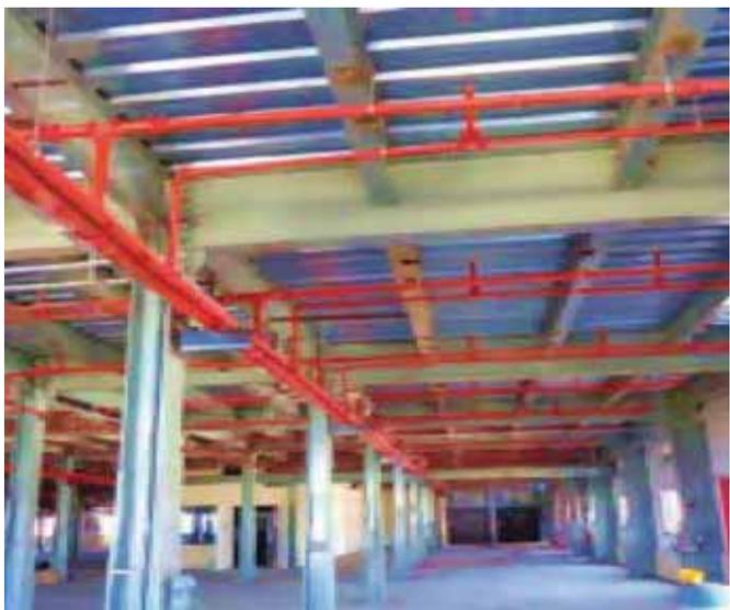
Automatic Foam Sprinkles System installed with QBD & IR3 detection
