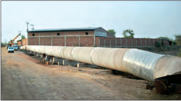
1700 mm dia x 10 mm thick M.S. Pipe Line with shrink wrap for curing for Raipur Augmentation WSS in Chattisgarh State
