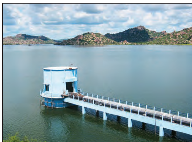
Intake well cum pump house for Mahabubnagar Water Supply Project, Hyderabad, A.P.
