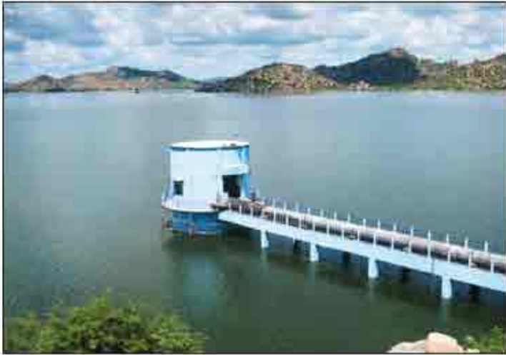
Intake well at Kolsagar
