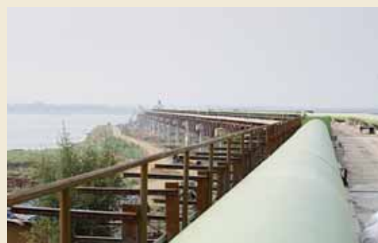
Twin Pipeline System, Santhaldih
