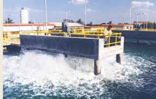
Tertiary Sewage Treatment Plant, Yelahanka
