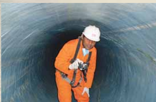
Sewer Rehabilitation Implementation
