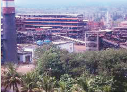
View of Sinter plant at Koppal
