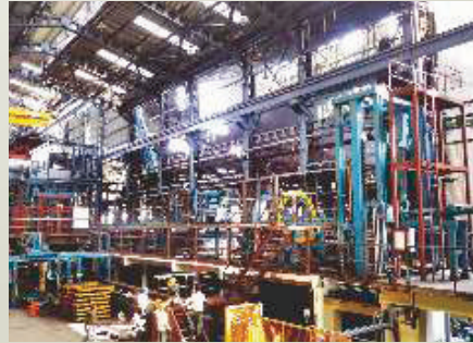
Moulding Line Under Installation at Koppal
