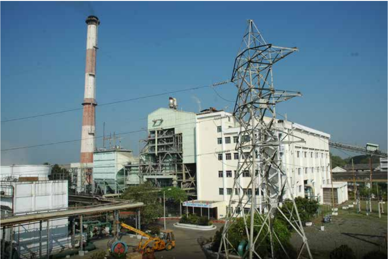
India's first co-generation power plant from sugarcane bagasse
