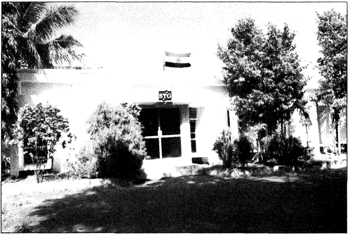
FRONT VIEW OF STG
