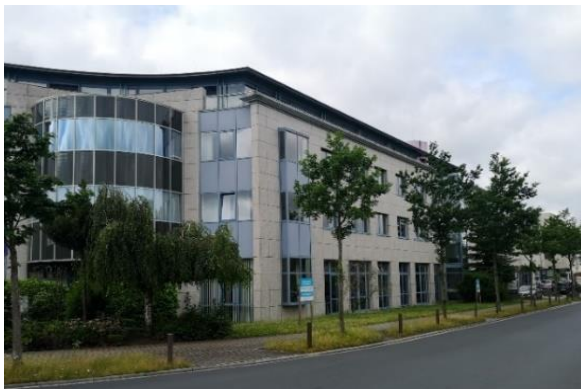
R&D Office, Germany
