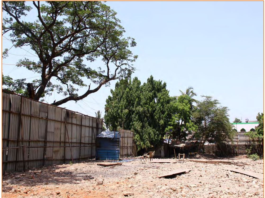
DEMOLITION OF STRUCTURE COMPLETED
