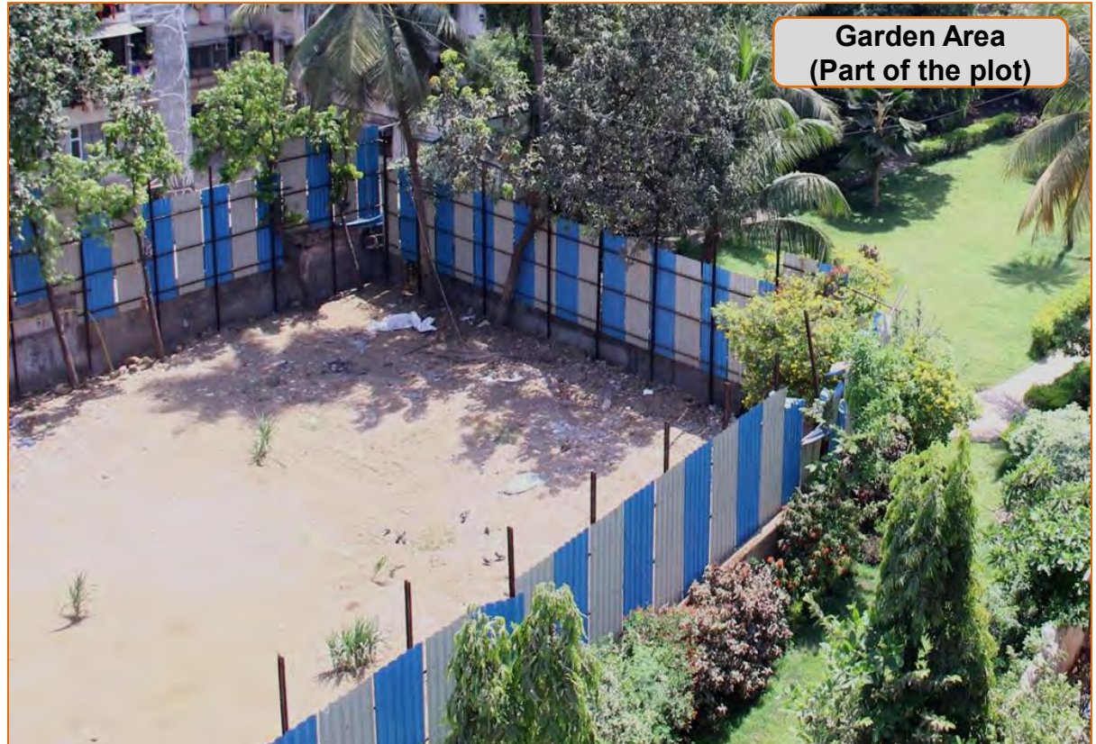
DEMOLITION OF STRUCTURE COMPLETED
