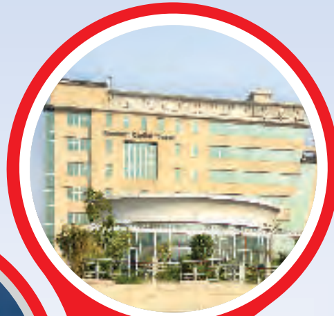
Parsvnath Capital Towers, B.V.S.M. (New Delhi) Actual Picture
