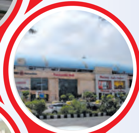
Parsvnath Mall, Akshardham Metro Station (Delhi) Actual Picture
