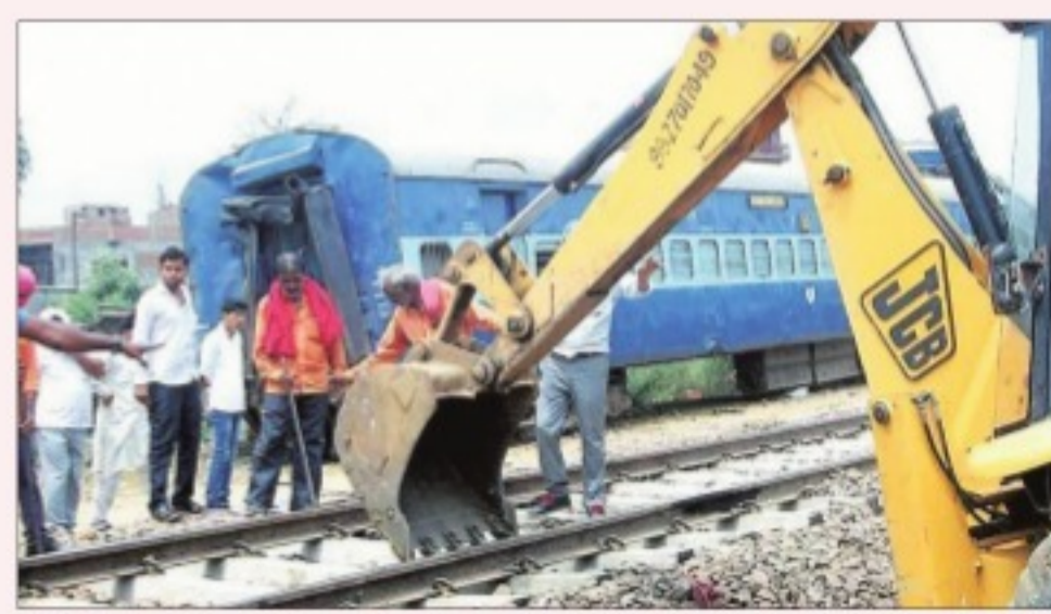
Workers repair the tracks at the derailment site
