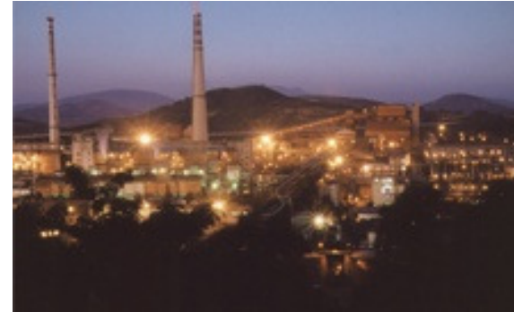
Alumina Refinery Damanjodi
