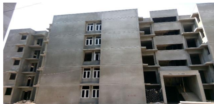
Happinest Boisar – Building B3 (Dec'15)
