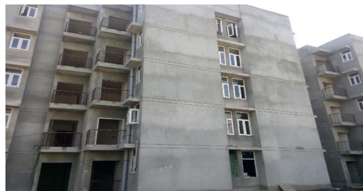
Happinest Boisar – Building J1 (Dec'15)
