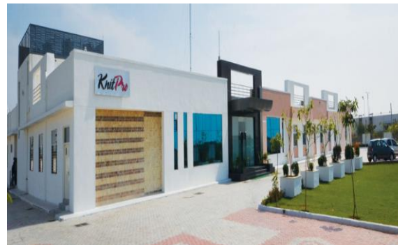
KnitPro facility in Engineering SEZ
