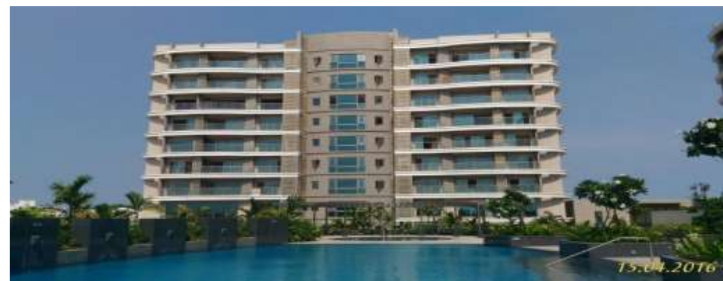
CREST TOWER A
