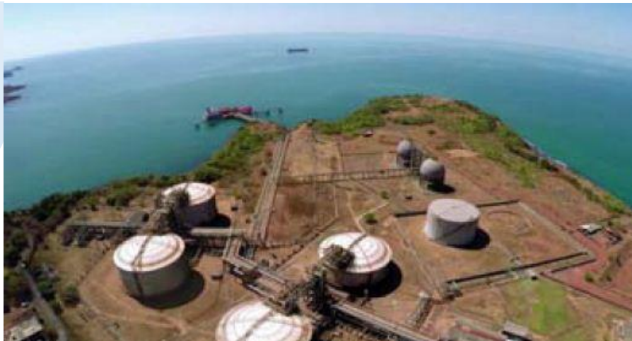
Storage tanks for raw material
