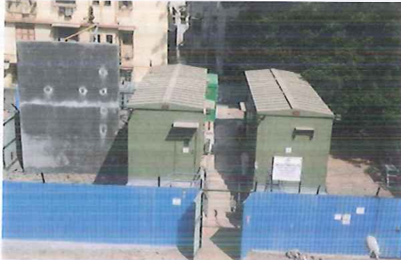
Tata Power's first Pre-fabricated 33/11 kV Power Distribution Centre
