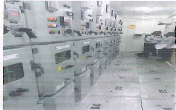
Tata Power's first Pre-fabricated 33/11 kV Power Distribution Centre
