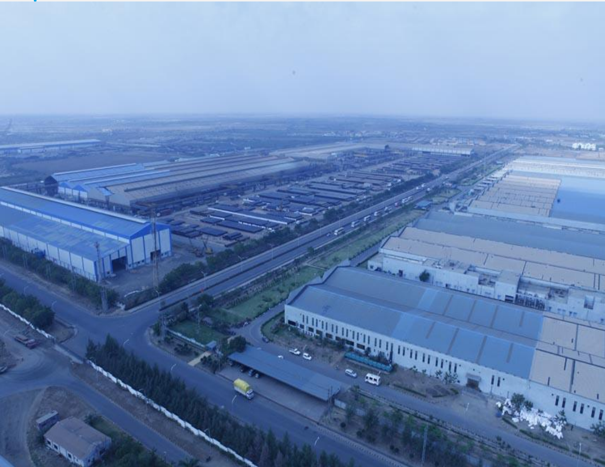
Aerial view of Anjar facility – spread over >1,000 acres with captive power generation
