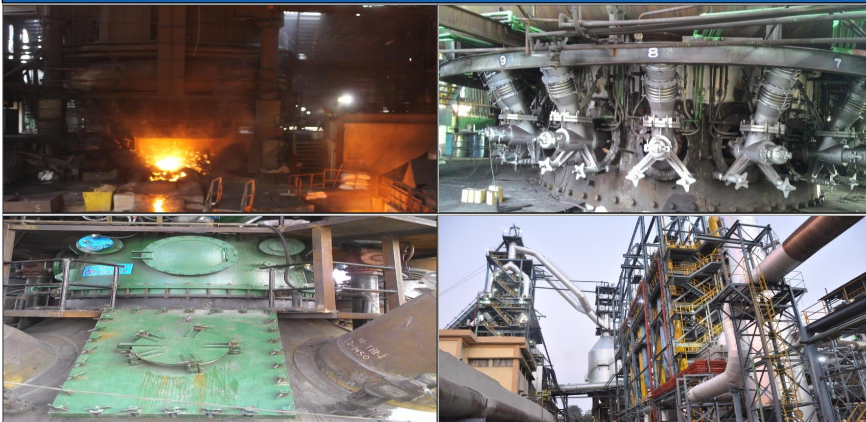
Blast Furnace reconstruction at Salem: re-commissioned in 4QFY16
