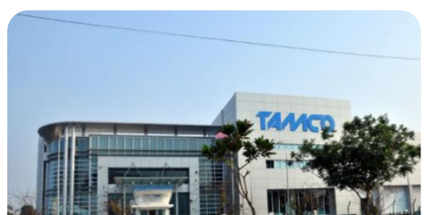
MV Switchgear Factory, Malaysia
