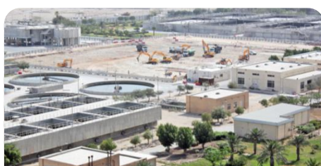
Water Treatment Plant, Doha
