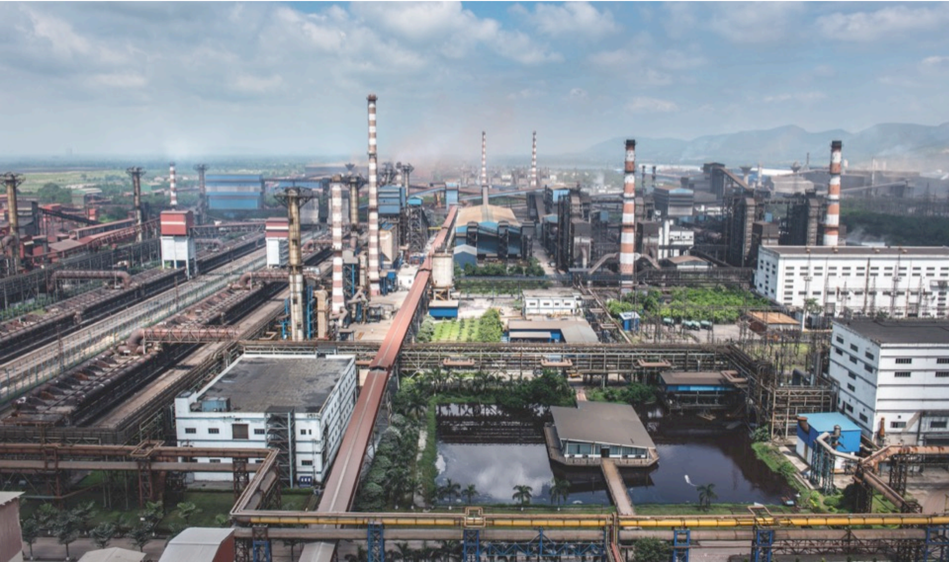
Aerial View of Raigarh Plant
