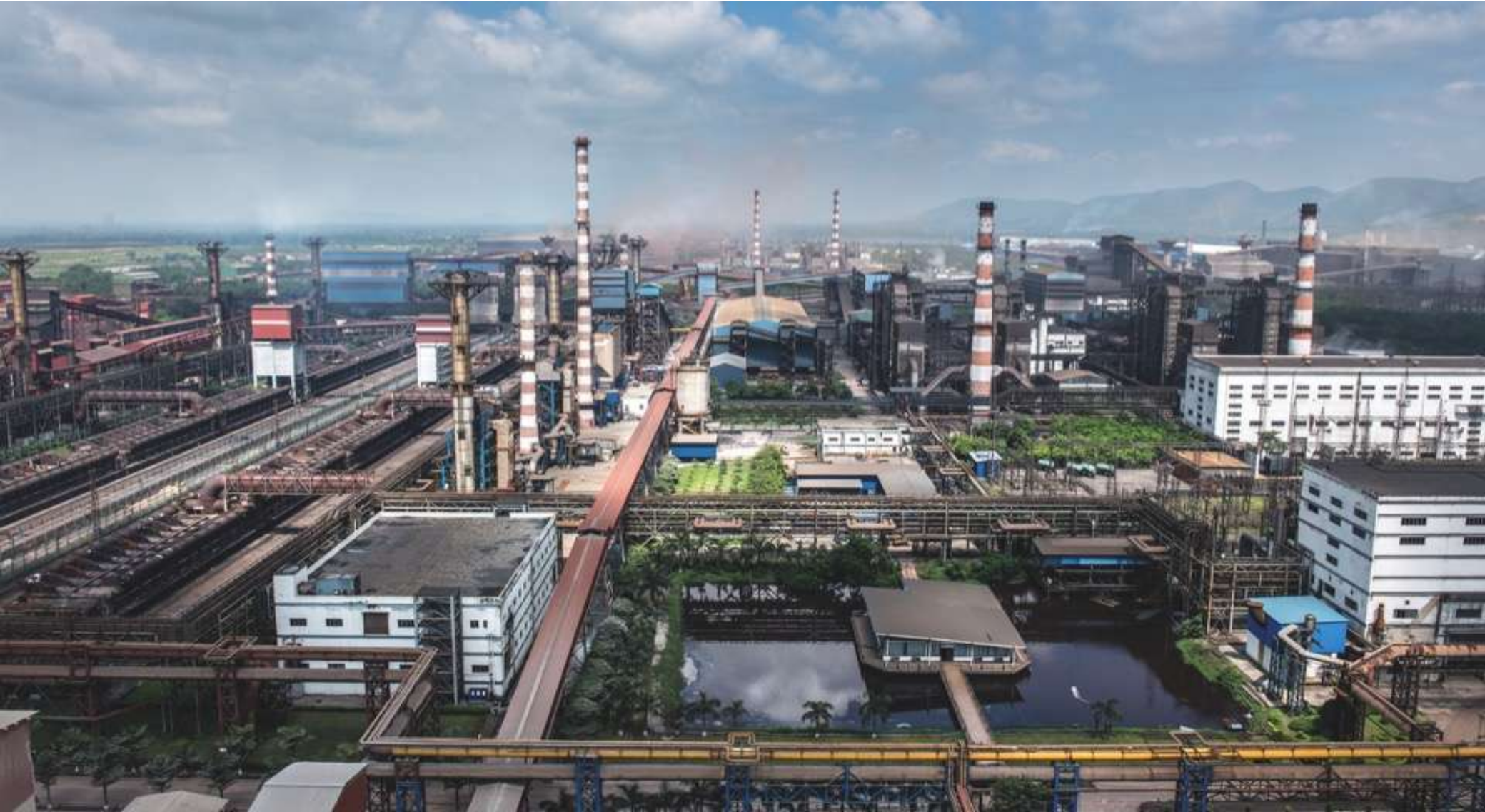
Aerial View of Raigarh Plant
