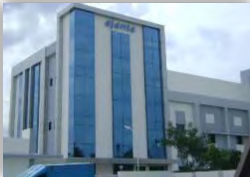
API Plant - Waluj
