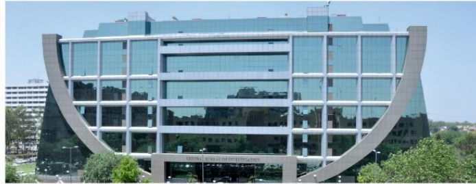
CBI HQ BUILDINGS, NEW DELHI
