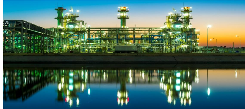
Rajasthan: Mangala Processing Terminal
