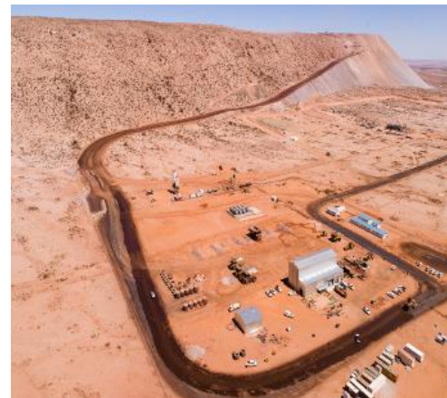
North access ramp including mining workshops
