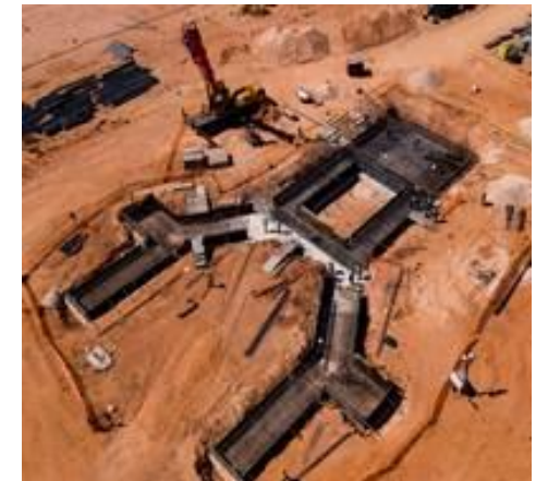
Civil footprint for the concentrator works
