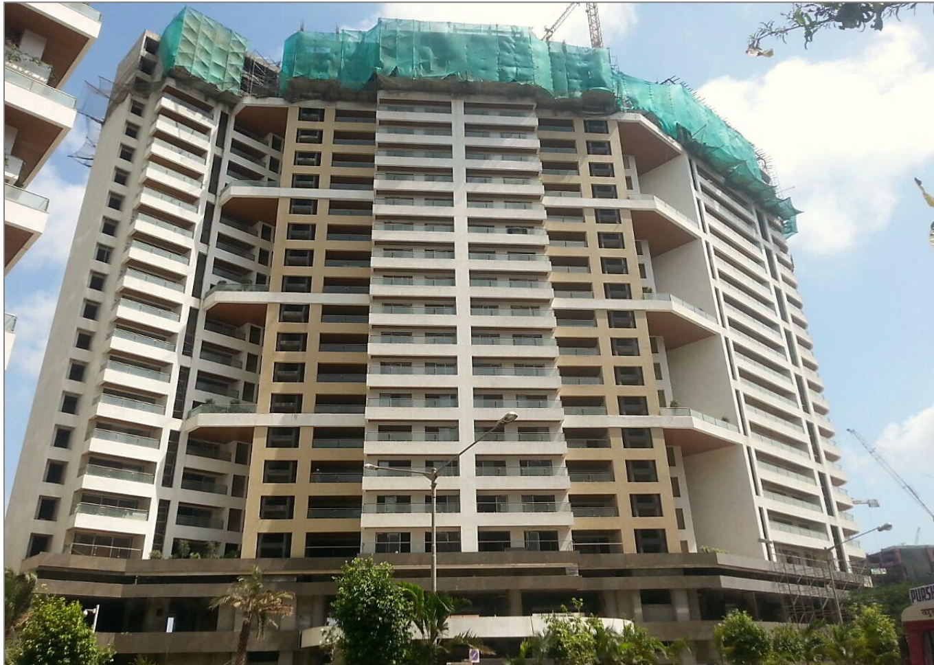
Final stage of RCC work-in-progress Finishing WIP
