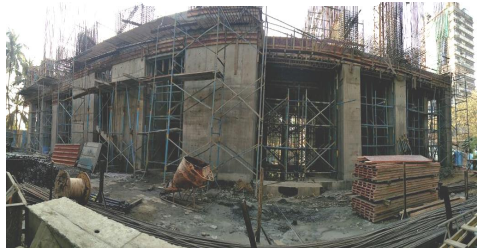
Tower C: 1 st slab completed
