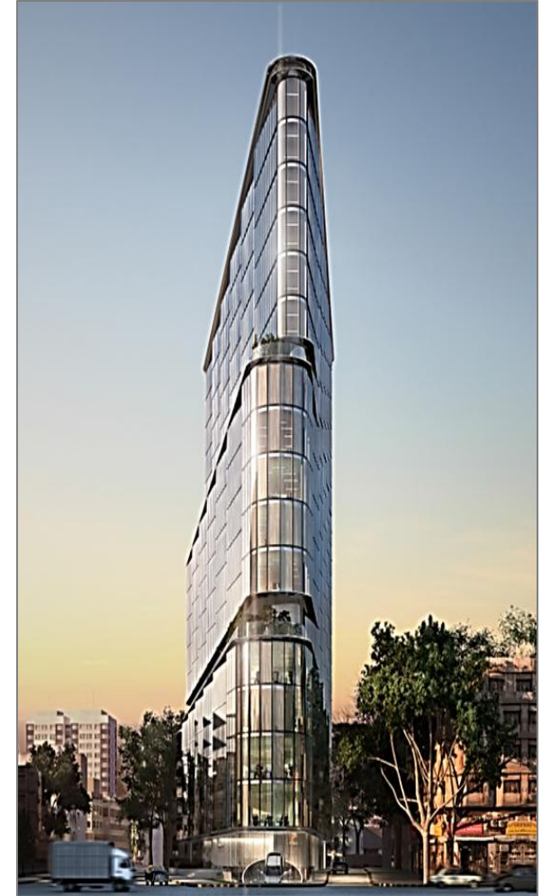
Sunteck Gateway 51, BKC Junction, Mumbai - Commercial
