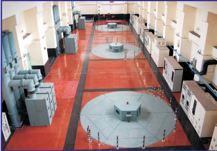
120 MW Sewa-II Power Station, (Jammu & Kashmir) - Machine Hall of Power House
